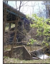
The East Branch Dam was constructed in 1933 to impound water for swimming at a YMCA camp. The dam is roughly 6 feet high by 40 feet wide and made of concrete. Over the years, the area behind the dam filled with sediment and now provides no recreation or other essential purpose.
